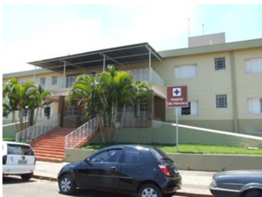
Fachada do hospital
